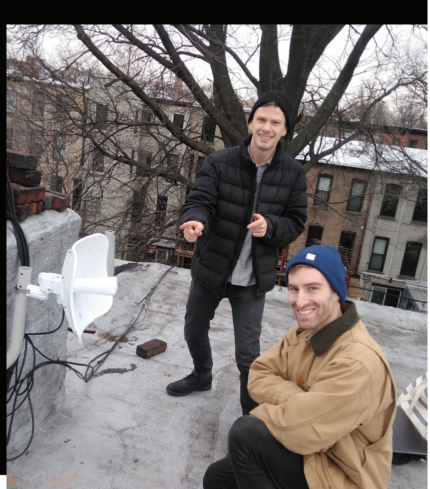
Volunteers successfully installing a Litebeam in Brooklyn.
